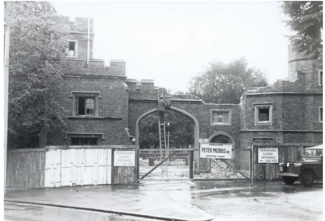
Demolition of the Lodge Gates in 1970, in line with the widening of Rickmansworth Road (old road alignment bottom left of photo)
